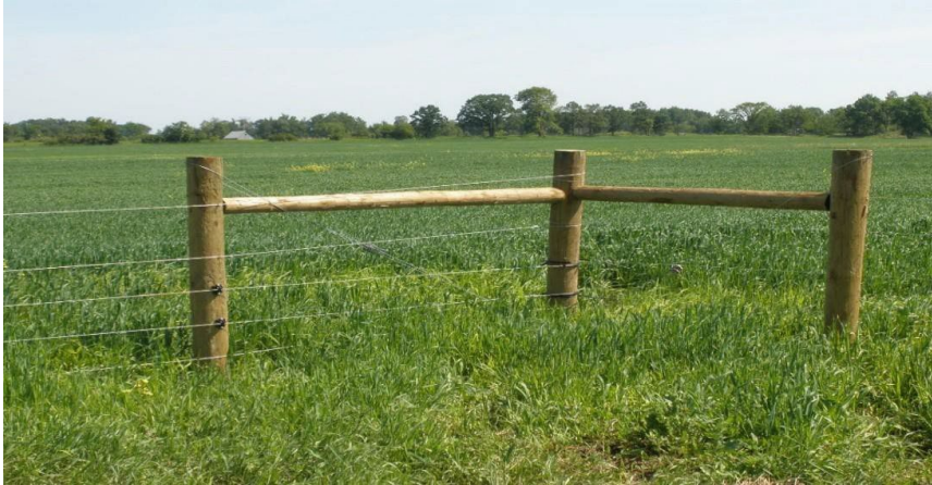
Photo 1. Power Fence. High Tensile Electric. Standard drawing located on page 4: Drawing Number MN-ECS-016.
